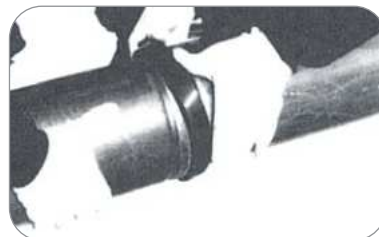
4. Slip on gasket to other pipe end
