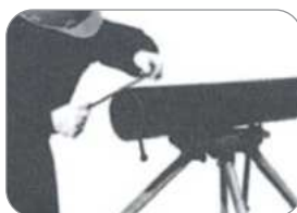
2. Smoothing pipe ends
