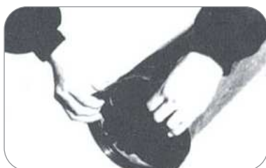
3. Slip on gasket to pipe end
