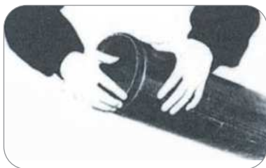
1. Inspect pipe ends for smoothness
