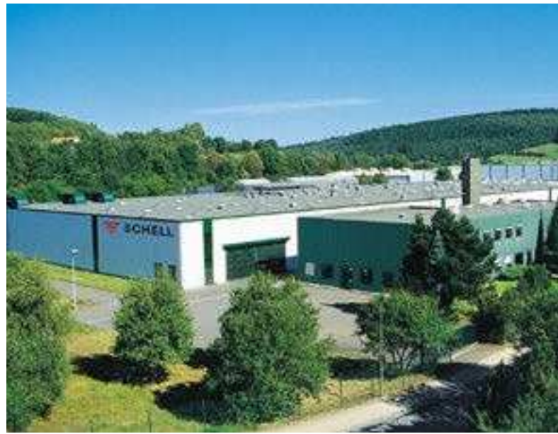
Plant 2 Production with logistics centre
